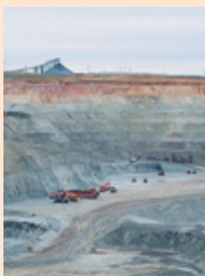
Pre-split drilling and blasting at Aktogay to preserve pit wall stability
